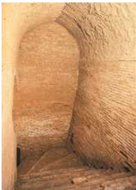
Ýerasty suw saklaýja girelge. Şähryslam. Entrance to underground water reservoir. Shaehrislam.
